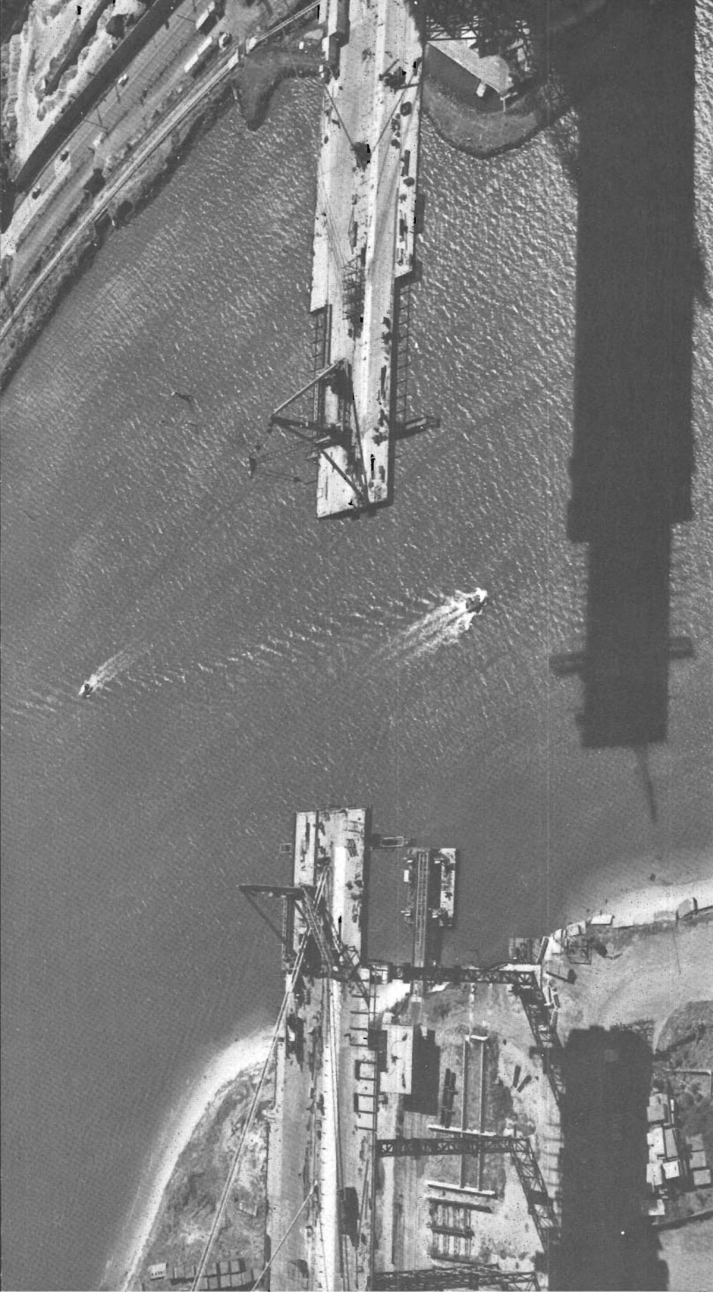
A dramatic aerial photograph of the West Gate bridge showing construction on the 336 metre main river span, December 1977.
